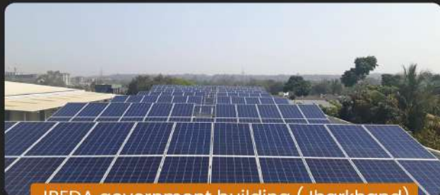
JREDA government building (Jharkhand)
